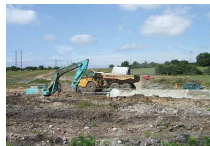
Work in progress at Smartcastle area
